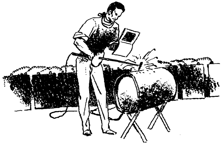
Welding with power from banks of batteries—1890
