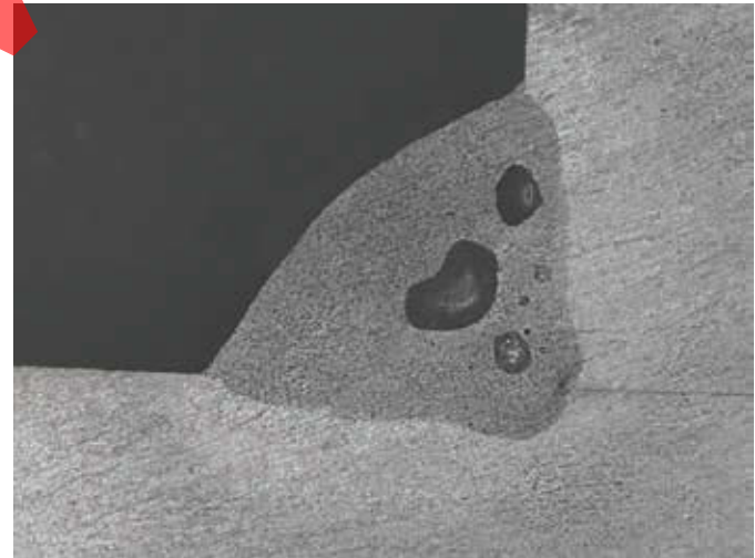
Figure 15 – Macro Etch Of Fillet Weld Showing Large Irregular Shaped Porosity.
