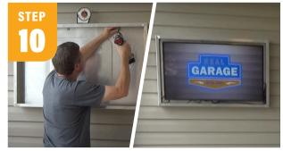
To hang the enclosure, put a couple of holes in the back to mount it to the wall. Also add another hole for the power cord.
