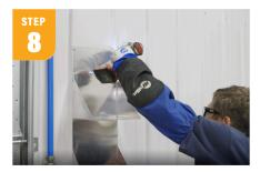
Mount the completed rack to the wall using a drill and sheet metal screws.
